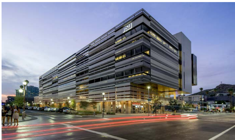
CAVC Building on College Ave, ASU Campus
