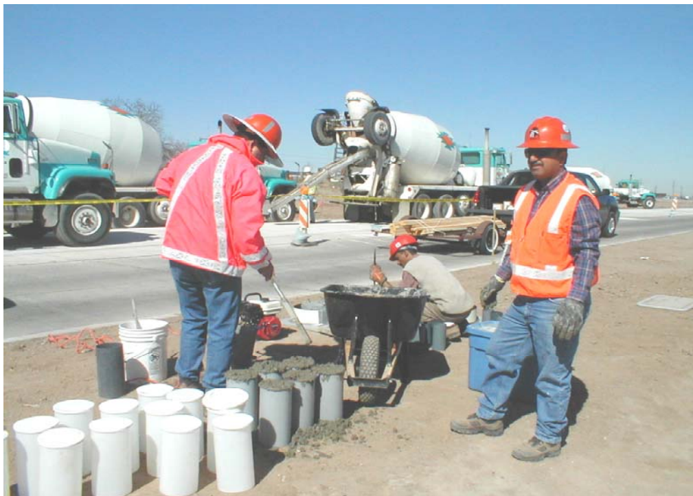
Figure 3.20. Collection of test samples from pavement sections
