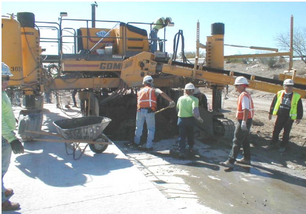
Figure 3.19. Concrete pouring in test section of pavement
