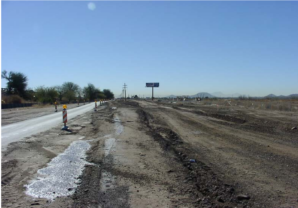
Figure 3.15. The access road prior to roadwork alignment
