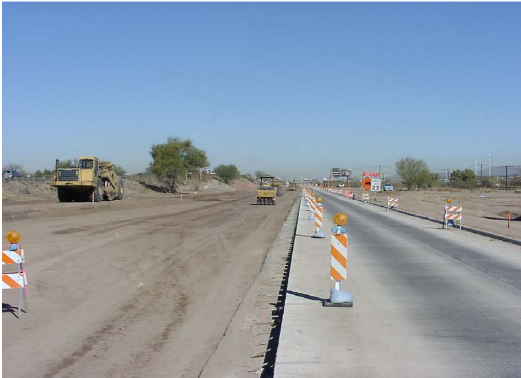
Figure 3.16. The access road during sub base preparation
