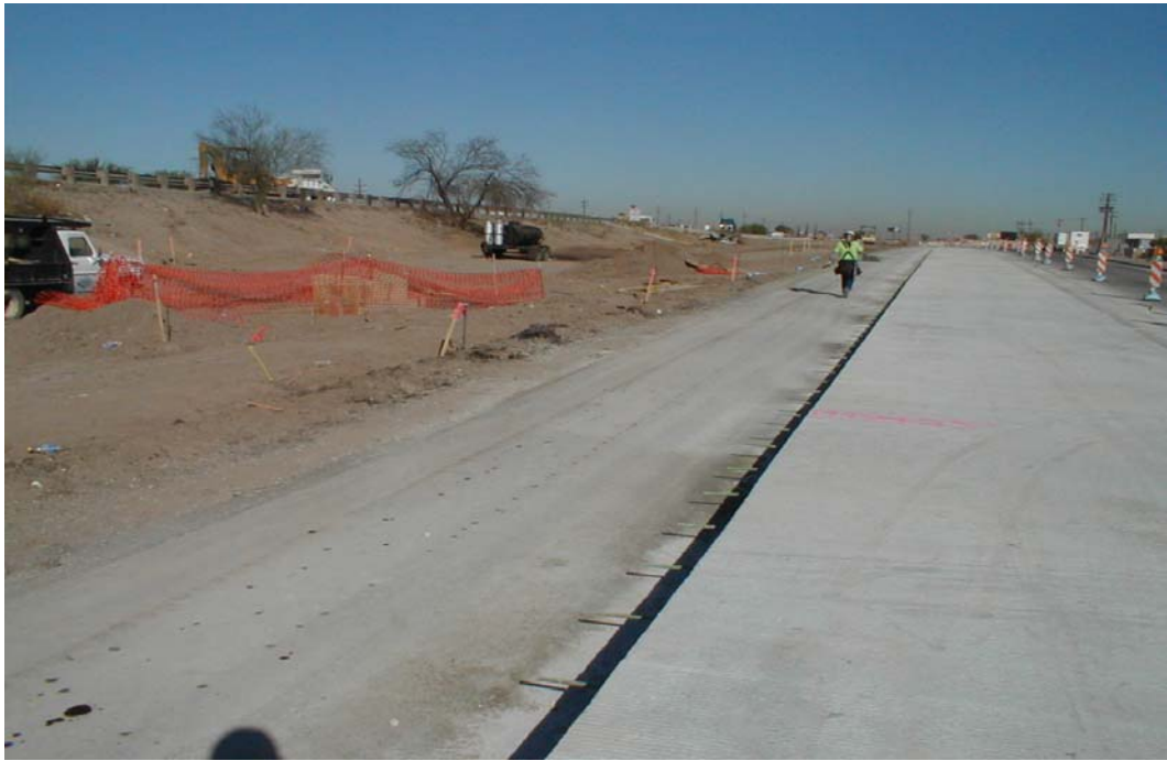
Figure 3.17. The completed sub-base prior to placement of concrete
