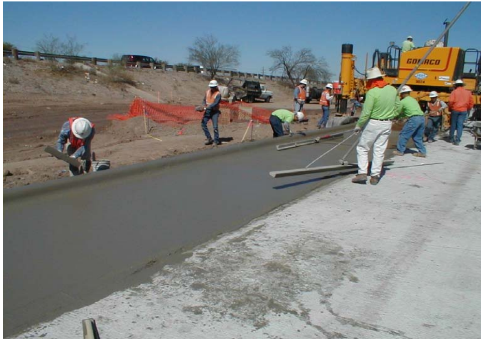
Figure 3.21. Test section of pavement during pouring of the high flyash mixtures
