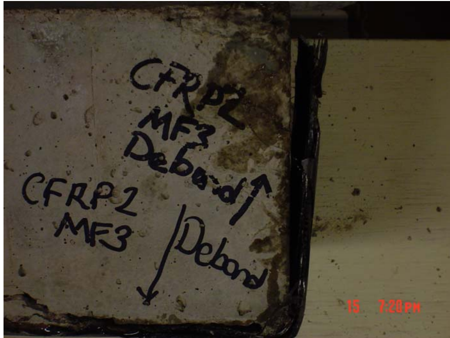
Figure 5.2.3.4. Debonding at the edges of the 2 layer CFRP reinforced concrete beam sample
